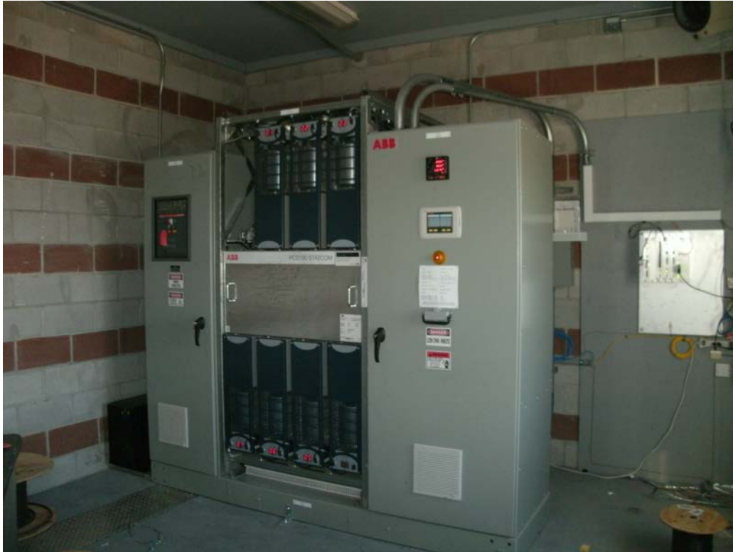
Figure 12.33. 300 kVAr SVC at the Bondurant, Wyoming, Site
