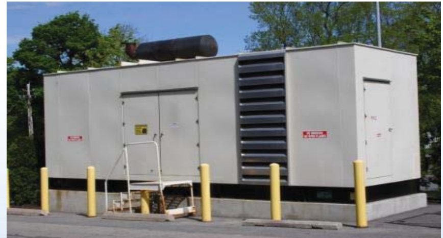
On-Site Back-Up Power Generators
